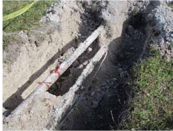
Figure 16 & 17 Lateral deformation of a pair of parallel pipelines due to underground earth movement detected by SCT™'s 3D mapping functionality.
