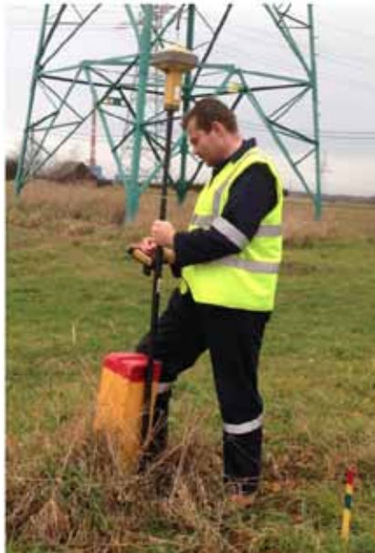
Figure 13 Electronic logging of location of topographical features above the pipeline route using UNISCAN's™ GNSS system.
